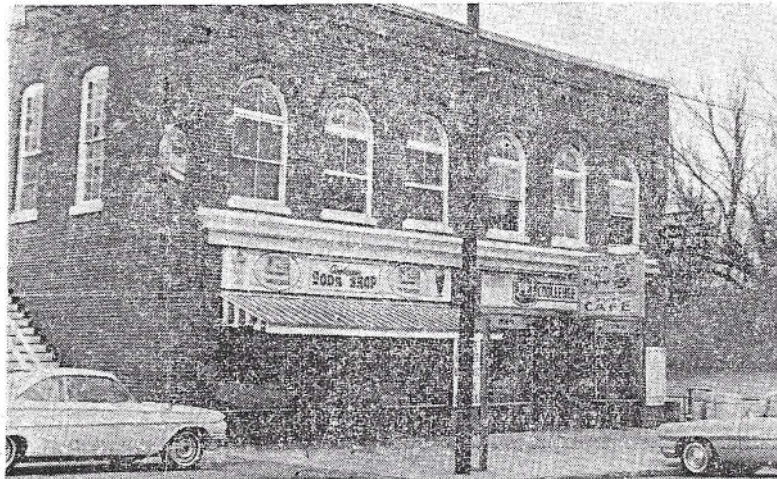
UNION HALL BUILDING — This building, on the east side of main street in downtown Cooleemee, reportedly is scheduled for demolition to make more parking facilities available. The only
